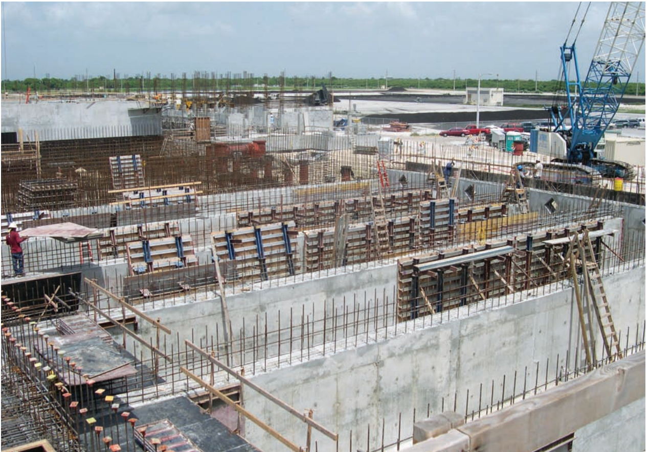
Miami-Dade Water & Sewer Department added Con mic Shield to specifications for new assets such as four 200-foot-diameter clarifiers.
