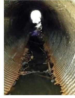
The CMP failed so completely along the invert erosion created a 3 ft. deep trench along the sewer bottom
