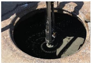
Manhole spincasting with Permacast system
