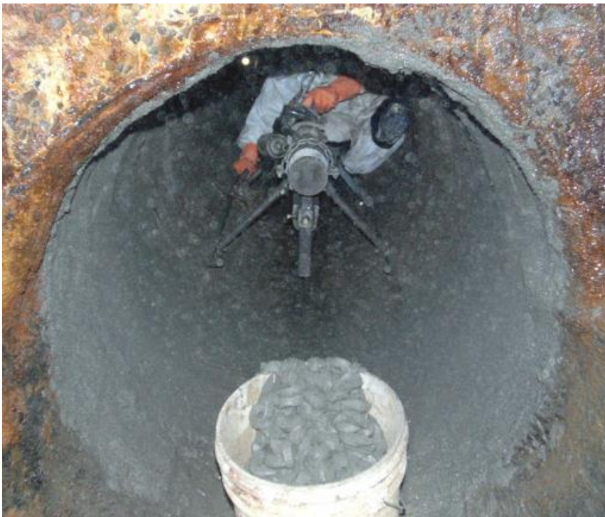
Spin-casting onto sheet steel inserts for fully structural rehabilitation of interceptor
