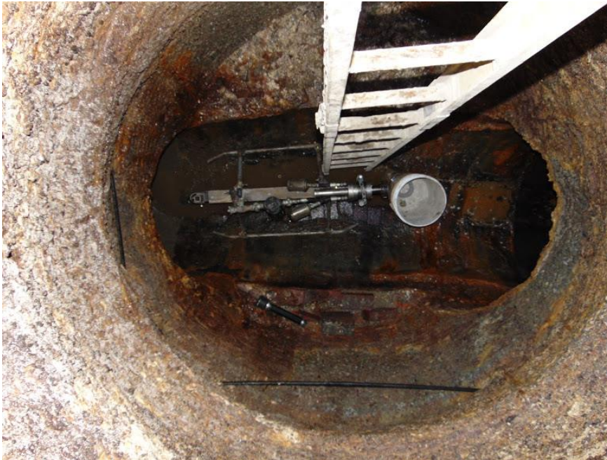
Manhole entry for rehab installation
