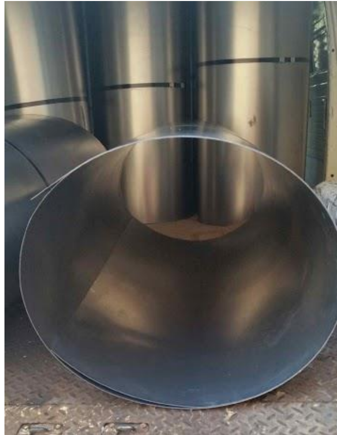
Custom sheet steel inserts to be inserted into failing interceptor
