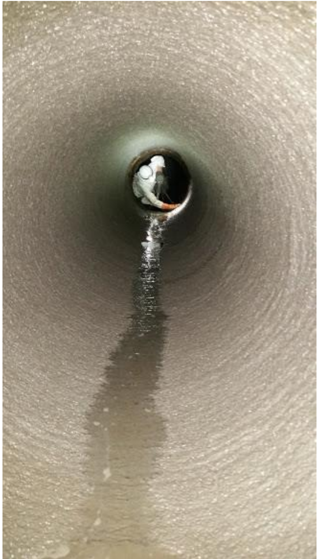
Fully rehabilitated interceptor
