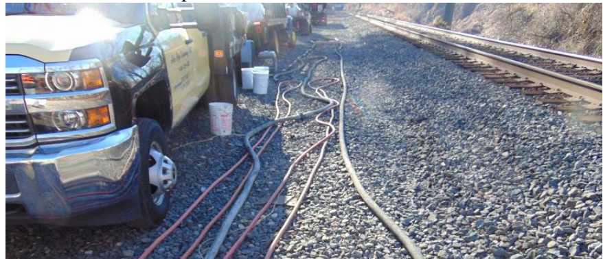
Interceptor site running parallel to railroad tracks and underneath two roadways
