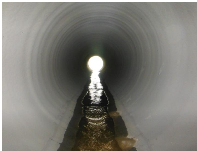
96" Round Culvert After Centrifugally Cast Rehabilitation
