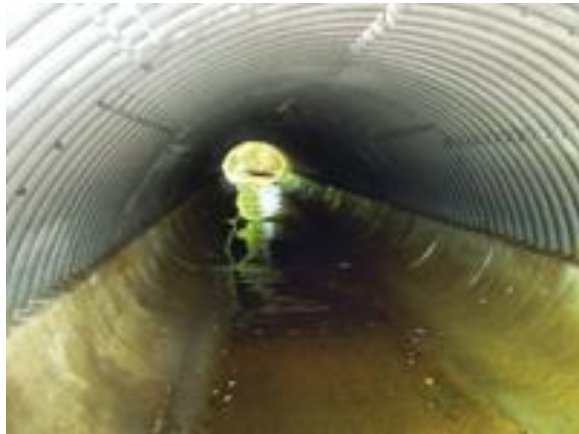
An example of a culvert with a paved invert
