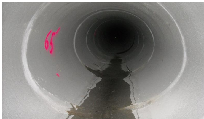
Rehabilitated pipe is smooth, seamless, structural, and watertight
