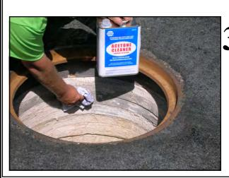
When air blasting is finished, an acetone wet wipe of the entire surface to be coated is recommended. This is to get a mechanical wipe of the surface, a wet wipe of the surface and a high flash point wipe of cementitious portion of the surface to evaporate any surface moisture in the non metallic portion of the chimney area to be coated with Flex-Seal Utility Sealant.
