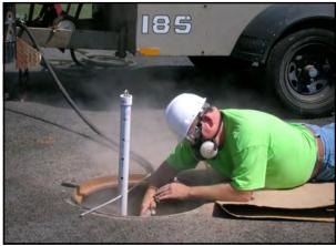
After sandblasting, blast the surface with clean air to remove any loose sand that may have been deposited onto the surface. The substrate surface **MUST** be dry and be free of loose sand.
