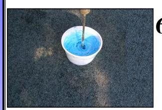
Use a power drill of at least 2500 RPM'S with a paint mixer attachment to mix A & B together. Blend the Flex-Seal Utility Sealant mixture using the drill-mixer with an up, down and around movement. This will insure a thorough air entrained mixture. IT IS VERY IMPORTANT TO MIX A & B TOGETHER THOROUGHLY. A uniform green color is required. After mixing the A & B materials it may be necessary to wait a few minutes for the mixture to reach its desired consistency.
