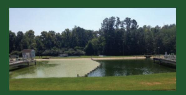
Picture: Wastewater Pond in Monroeville, AL separated with water curtain. Left side of pond remained untreated, right side of the pond was treated with High Volume Floating Aerators and Floating Mixers.
