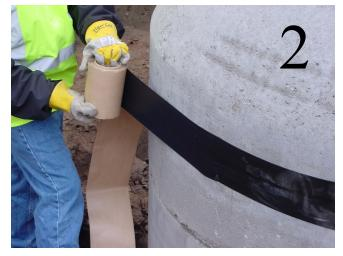
2. Remove the first foot of paper backing from the mastic. Center and place the Gator Wrap® around the joint. Continue to remove paper backing as you apply the Gator Wrap to the entire structure.
