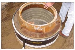
2 Stretch the Infi-Shield® Uniband over the casting and position it so that it will seal from the top of the casting frame's flange to the top of the cone section. Be sure that the inspection tap is at the top of the seal.
