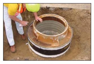
B Covering the entire adjustment area, fold back the top and bottom mastic portions of the seal. Apply the aerosol primer on the casting flange and top of the cone where the mastic will bond. Allow a few minutes for the primer to dry and become tacky.
