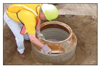
Clean the flange of the casting frame and the top 5-inch area of the cone of the manhole with a wire brush and a whisk broom. Both areas must be clean and dry.
