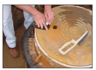
Clean a 5-inch area on the cover with a wire brush. Position the inspection tab on the side of the casting frame and onto the cover. Remove the protective tape from the mastic on the free end of the inspection tab and fasten the inspection tab onto the cover tapping it into place with a rubber hammer.
