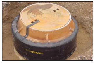
Back fill. Now you have a permanent seal between the manhole frame and the cone, including the entire adjustment area.
