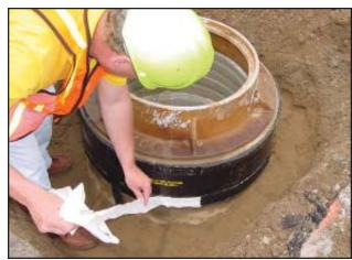
Remove the protective tape from the non-hardening butyl mastic strips.
