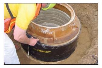
Fold the seal back onto the structure. Press the sealing surfaces together, bonding the Uniband to the flange of the manhole casting frame and the top edge of the cone. This creates a seal over the entire adjustment ring area.
