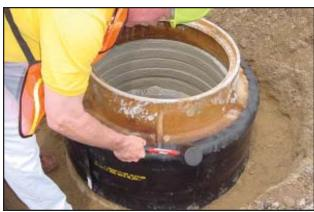
Now using a rubber hammer, tap the sealing surface area.
