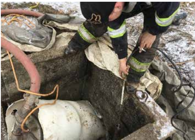
Raising liner skin temperature at A-side using Propane torch
