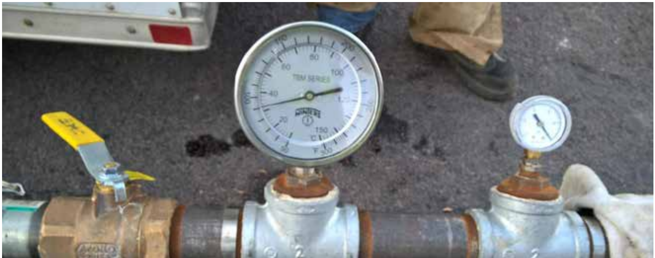
B-side control station monitoring temperature and pressure during expansion /cooling stage
