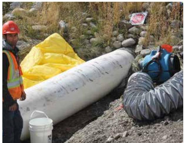
Liner expanded on A-side
