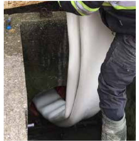
NovaForm liner pull head entering culvert
