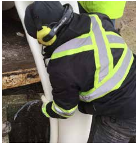
NovaForm liner pull head entering culvert
