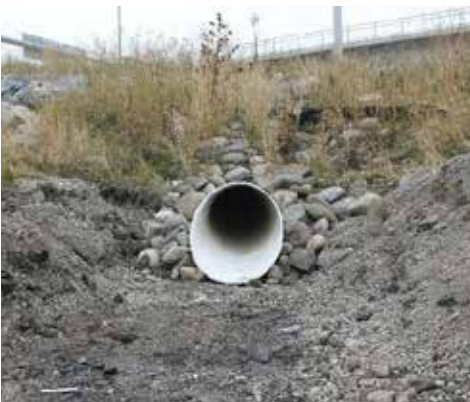
Finished and Trimmed NovaForm Liner (at outlet)
