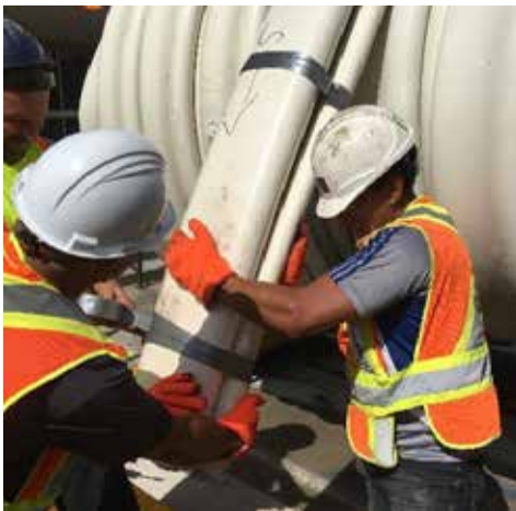
Liner pull head preparation (folded liner)
