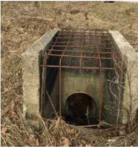
B-side catch basin looking upstream to A-side
