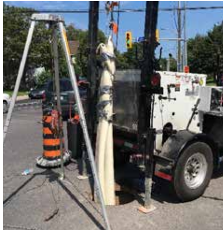
NovaForm liner exits at B-side manhole
