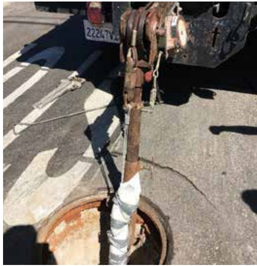
Liner emerging from B-side manhole
