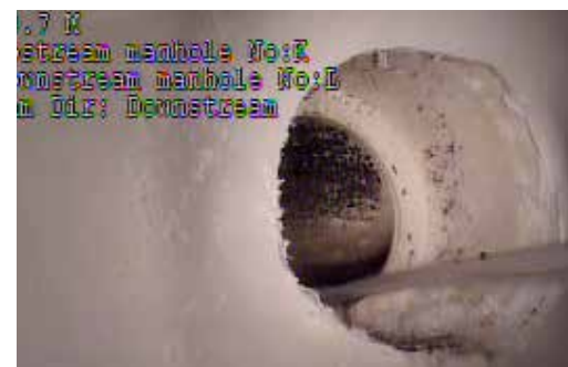
Active service that has been reinstated via robotic cutter
