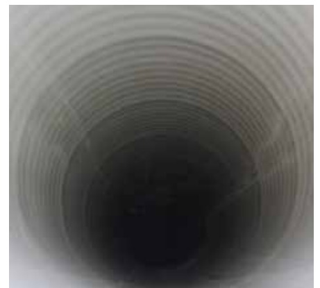
Inside of finished liner (at outlet)
