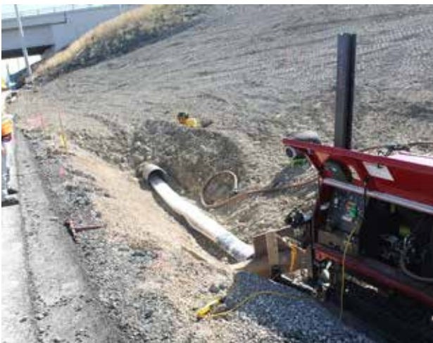
NovaForm liner pulled through to B-side
