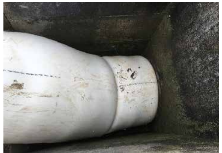
Liner expanded on B-side (flared)
