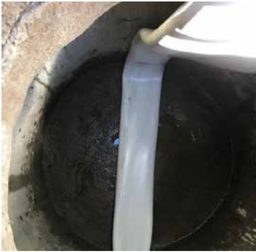
Liner pulled through at A-side manhole
