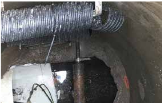
Finished and Trimmed NovaForm liner (at intermediate manhole)
