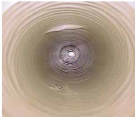
Inside of finished liner (at 100m)
