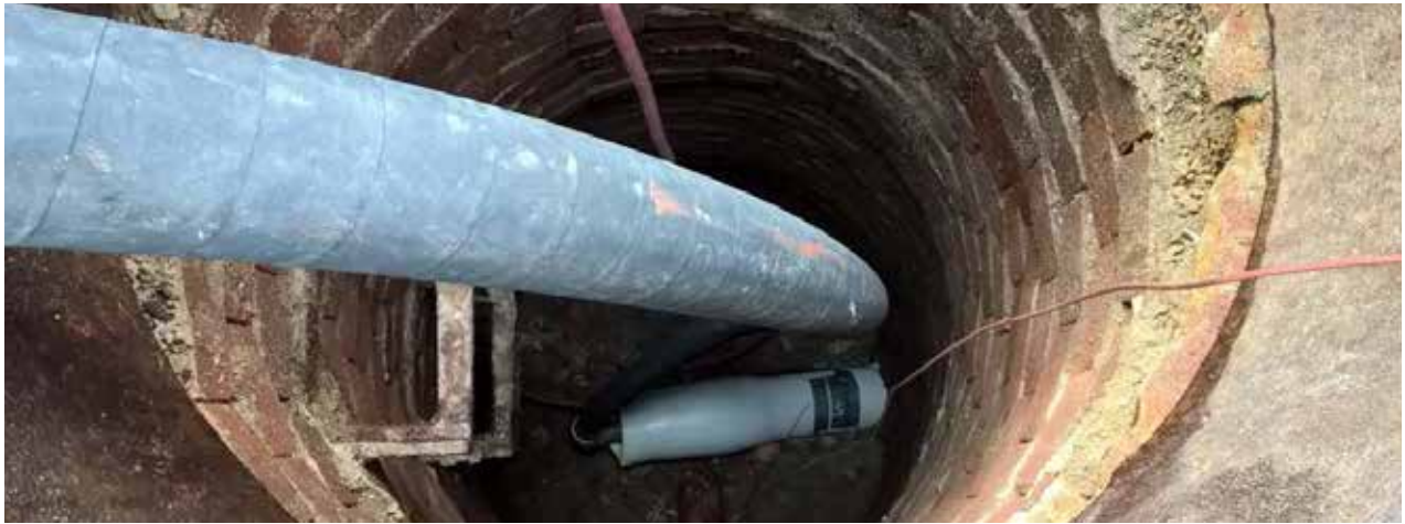
Thermocouple taped to liner on A-side for monitoring of temperature during processing
