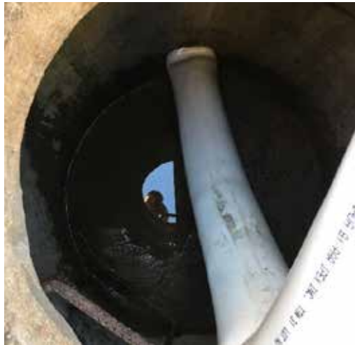
Liner starting expansion at A-side
