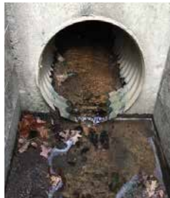
B-side invert (before)
