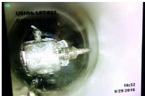
CCTV snapshot of reinstating service lateral via robotic cutter
