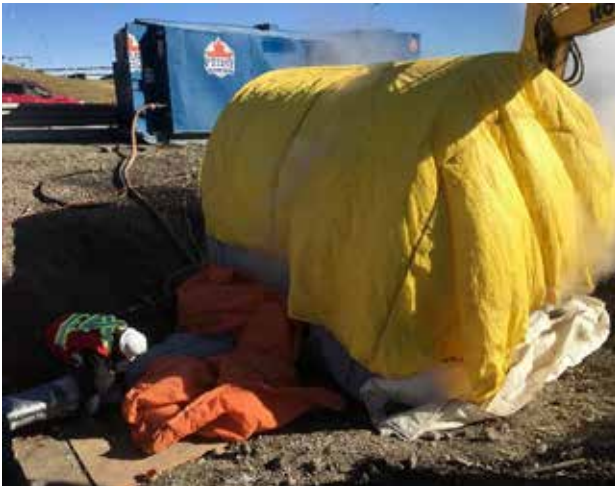
Liner conditioning under tarp on A-side
