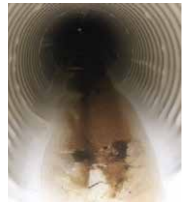
B-side invert (after)
