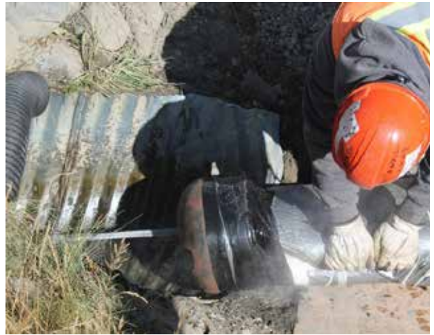
NovaForm liner pull head entering culvert
