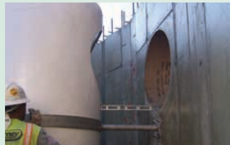
Strapping detail on Vortex unit, Buckeye, Arizona.
