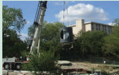
Offloading a Vortex Top Form.
