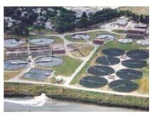
Lincoln, NE has over 1,000 miles of sanitary sewer lines and 16 pumping stations that keep the wastewater flowing to two municipal wastewater treatment facilities that treat up to 25 million gallons of water per day.
