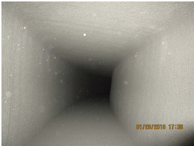
Radiused rectangular channel after lining completion
