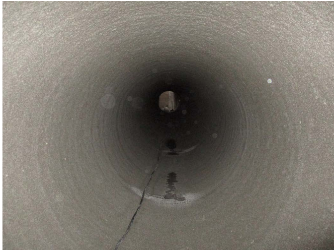
Circular channel after lining completion
